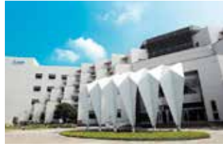
Tainan Plant (Diamond-rated Green Building)
